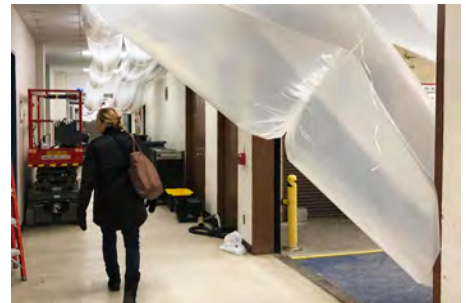
Large machines pumped super dry, 3% humidity air into the building for several weeks to dry out plaster and prevent the formation of mold.
